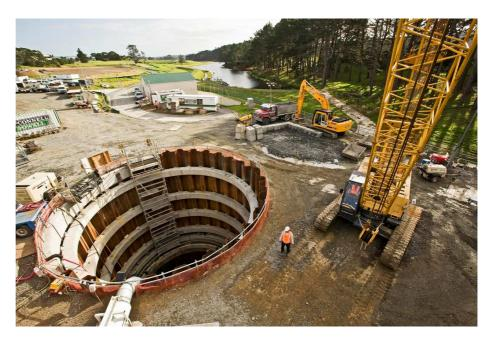
Figure 2 - Sheet piled shaft excavation during construction for the Rosedale sewer tunnel, source - TunnelTalk.com.
